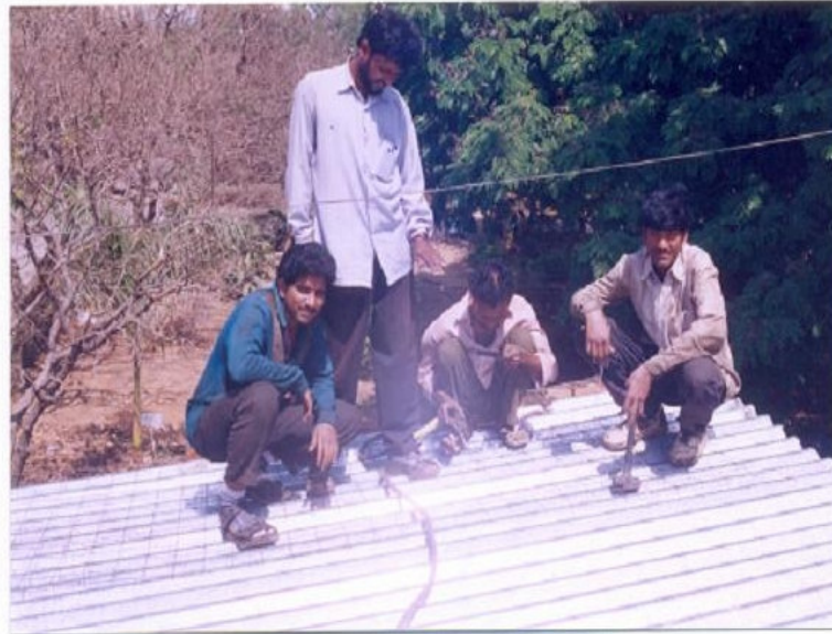
TEMPERATURE & SHRINKAGE REINFORCEMENT (WELDMESH TACK WELDED TO DECK SHEET)
