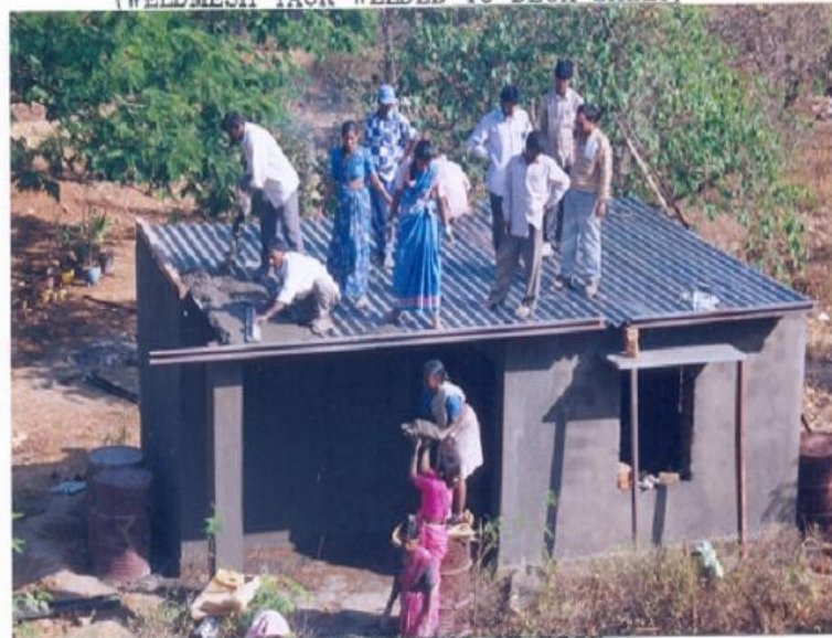
INSITU CONCRETING OF ROOF
