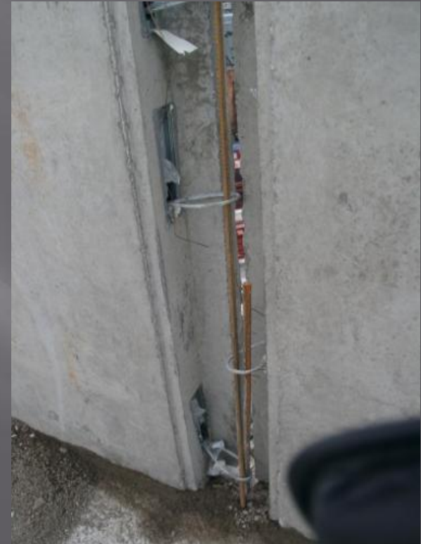
External Wall Connection - Loops and vertical Bar
