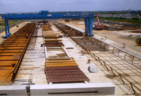
MOVING REBAR CAGE INTO CASTING BED
