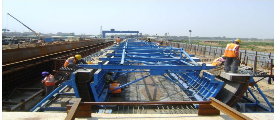
CAST FULL SPAN U- GIRDER ON CASTING BEDS
