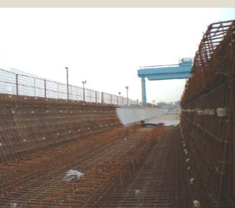
PRE-TENSIONING ARRANGEMENT
