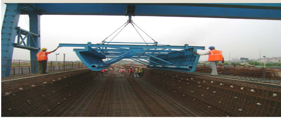
CAST FULL SPAN U- GIRDER ON CASTING BEDS
