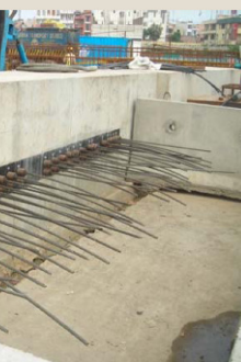
PRE-TENSIONING ARRANGEMENT
