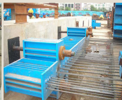
PRE-TENSIONING ARRANGEMENT
