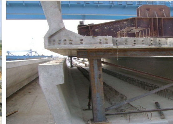
STACKING OF FULL SPAN U- GIRDER
