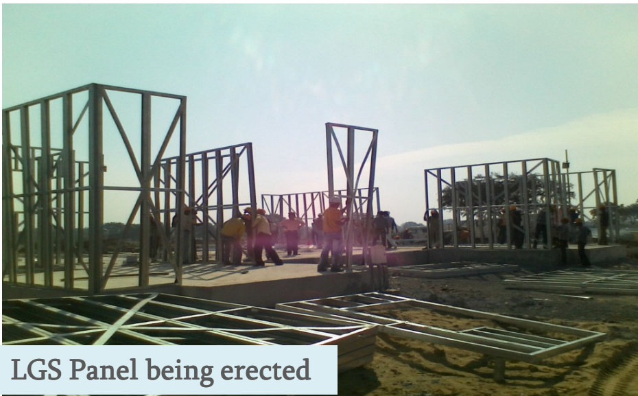
LGS Panel being erected
