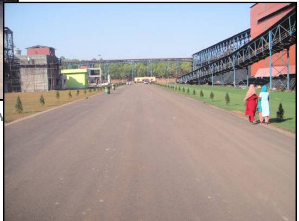
Bitumen layer on base layer built with JGRS Barbil
