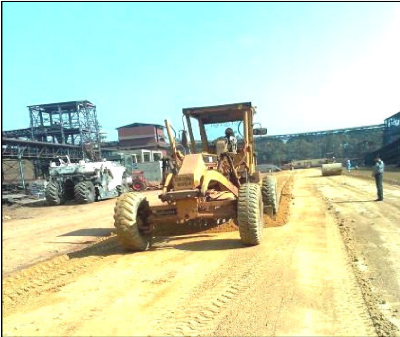
Performing a final cut using a Grader
