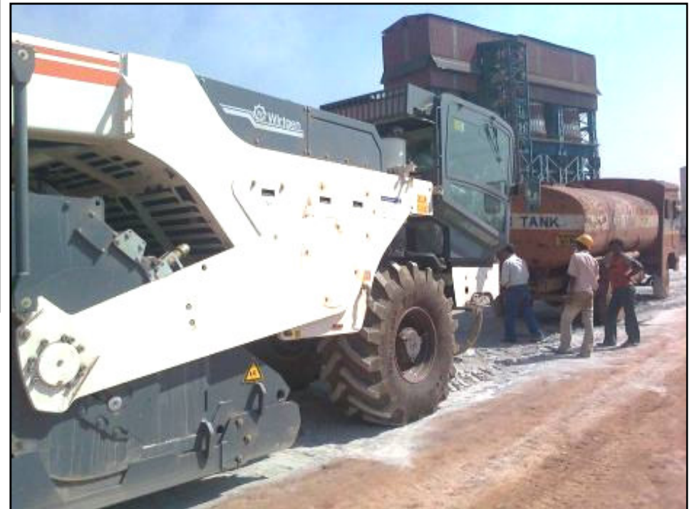
Recycler mixing JGRS with soil
