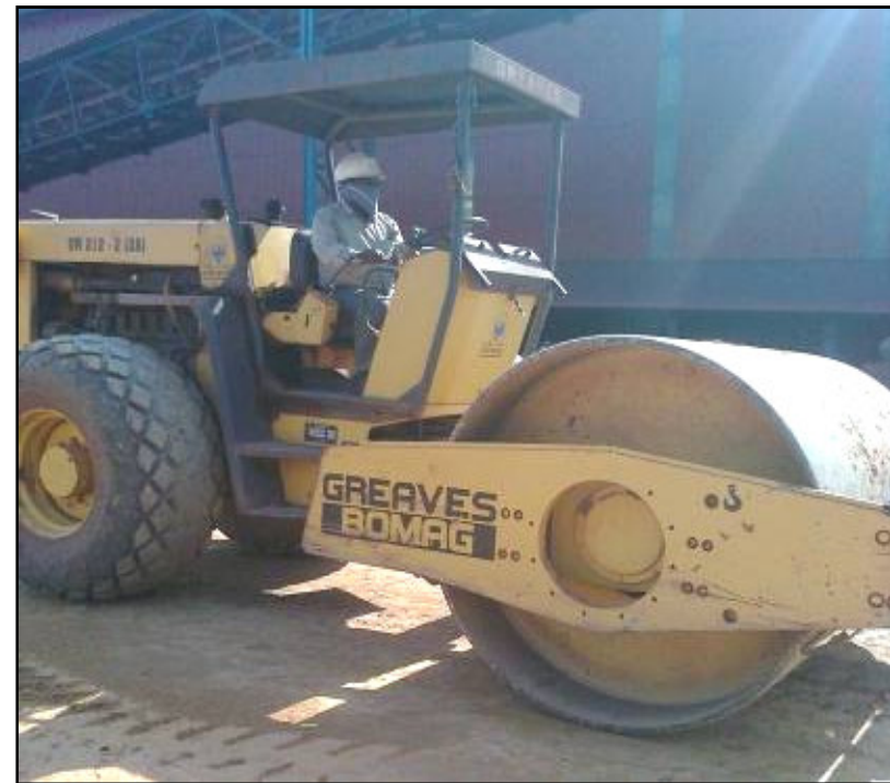
Compacting the surface with a Vibratory ro
