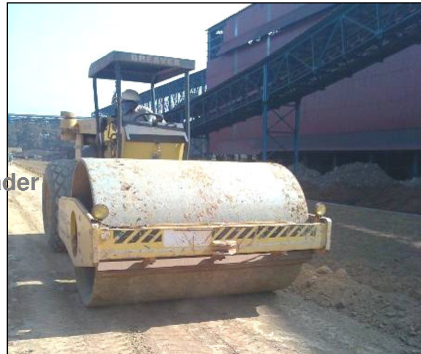
Smooth rolling done on final surface
