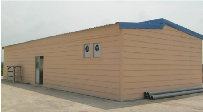
Site office for Brick plant, Raigarh 1500Sft:
