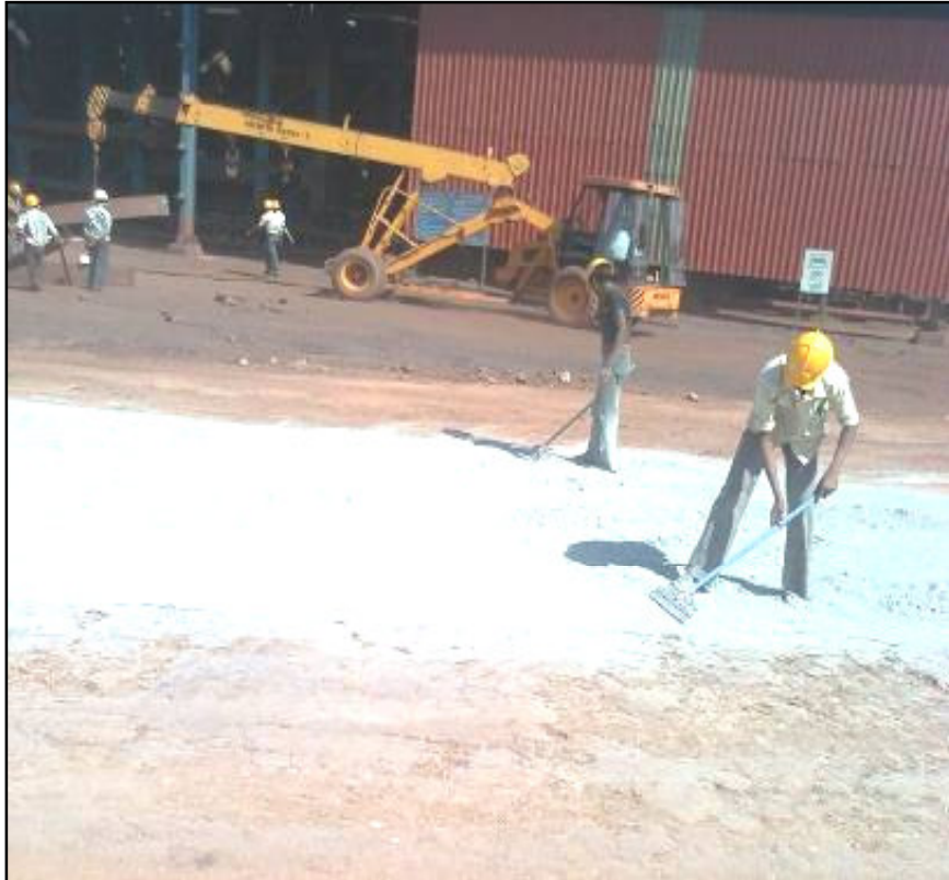
Spreading of JGRS
