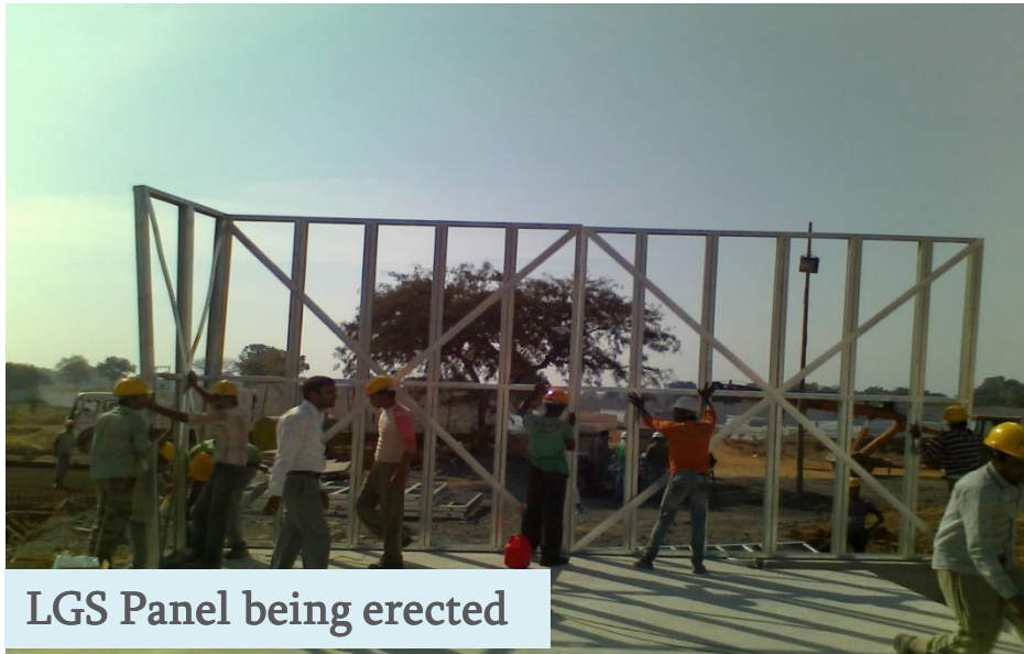
Installation of LGS panel
