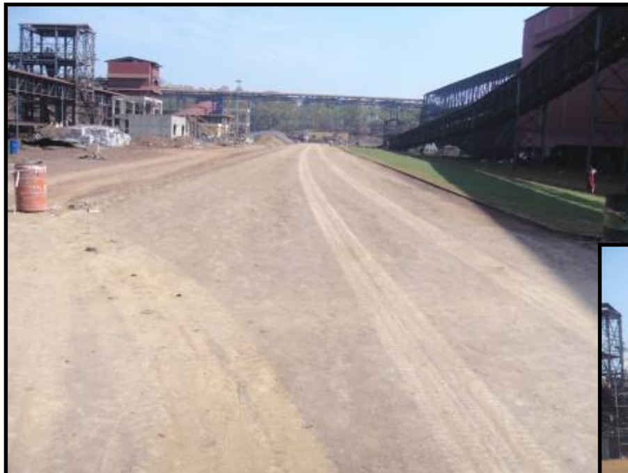
Finished surface of base layer built with JGRS Barbil
