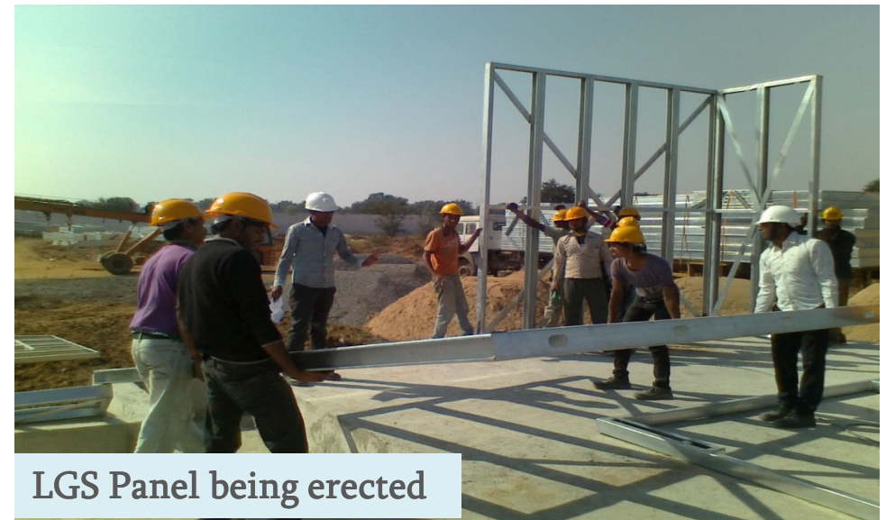
Installation of LGS panel
