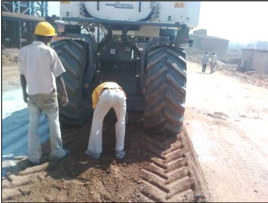
Recycler mixing JGRS with soil
