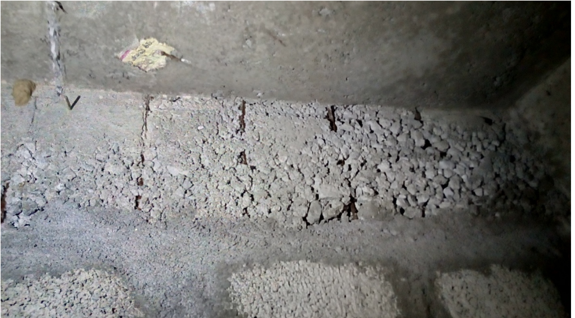
Severe honeycombs and Reinforcement exposed in roof level beam
