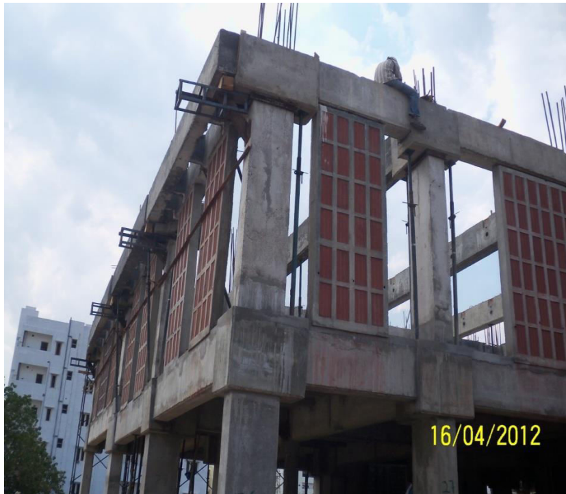
Precast walling with Hollow Terracotta block
