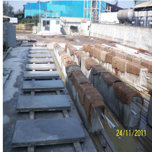
Connectors were welded on top of beam
