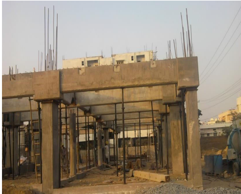
Erection of Stilt floor Individual Joists and stone panels
